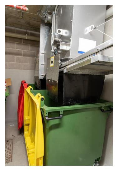
A service room should be provided on each floor of the development to allow access to the waste chutes and allow for materials that should not be put into the chute (e.g. FOGO material, large cardboard boxes, broom handles) to be stored for manual collection. Chutes should not open onto any habitable or public space.
