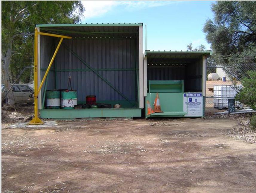
Picture: Used Oil Drum Storage Unit and 4,500L storage tank at the Shire of Williams.
